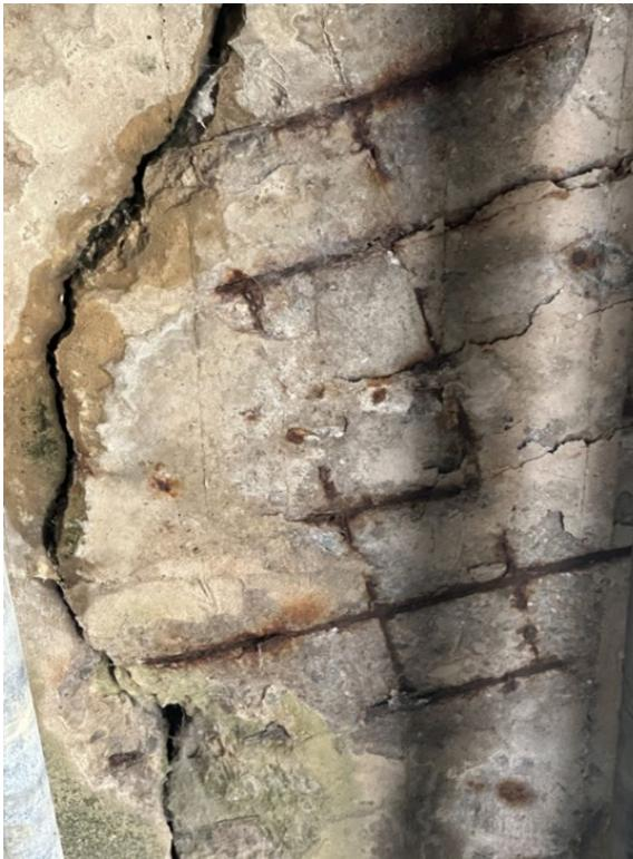
Concrete spall and cracks
