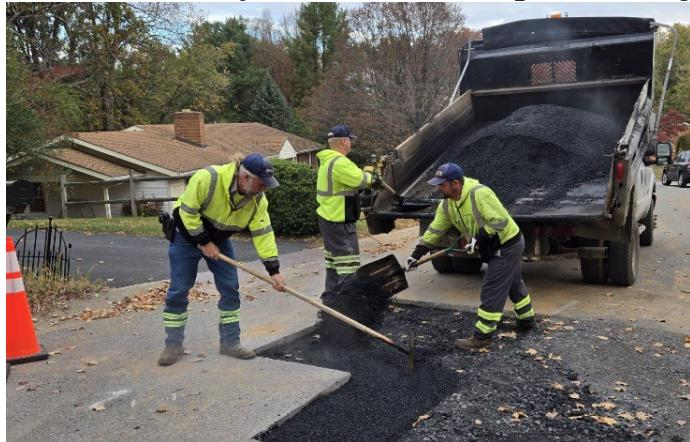
This photo is the Public Works asphalt paving crew in action, as led by Bobby Back, repairing a utility cut from a recent water main break. While other utility owner's (such as gas company, power company, etc.) are responsible for the restoration of their utility cuts, Public Works is responsible for their own cuts. Pavement restorations can stem from utility repairs, breaks, new services, or even just everyday street wear and tear or potholes.
